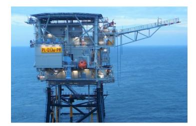
An existing oil and gas platform off the Dutch coast is being converted to the world's first offshore hydrogen platform. Electricity generated by offshore wind turbines will be used to convert seawater into demineralized water and to power a 1 MW electrolyser producing clean hydrogen.
